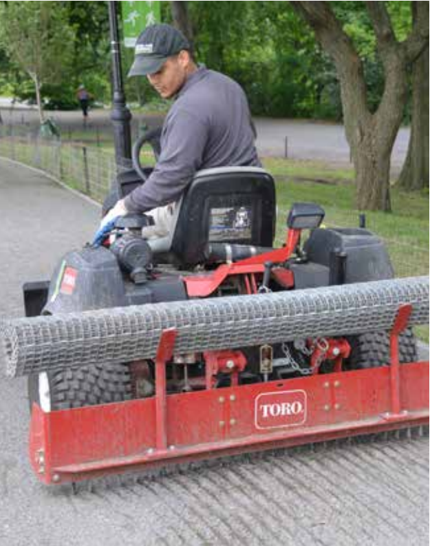
Gabe Hernandez incorporates new millings into the track.
